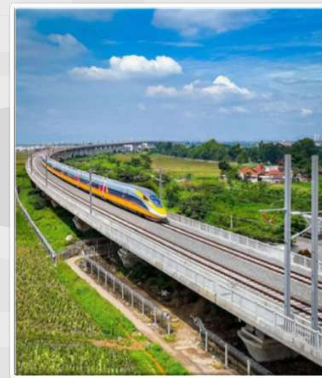
High Speed Railway Contractor Consortium Jakarta – Bandung High-Speed Rail
