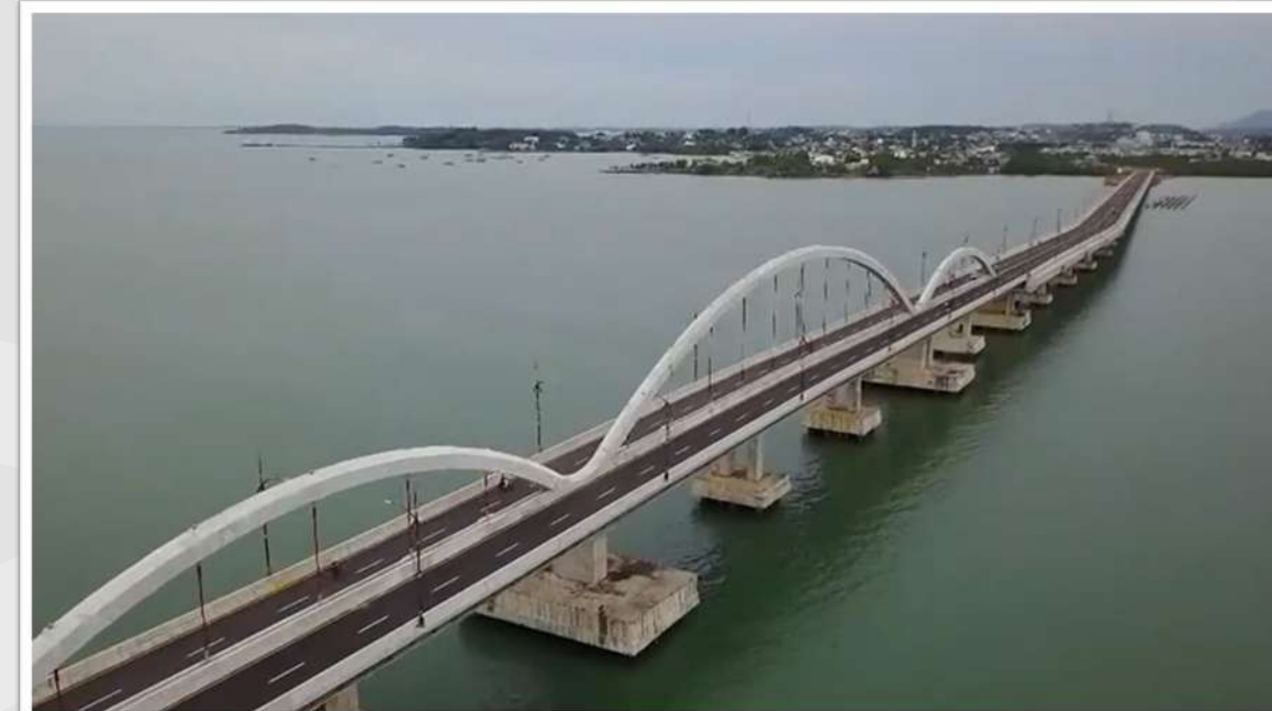
PT Wijaya Karya (Persero) Tbk Bored Pile Works for Dompok Bridge Construction Project
