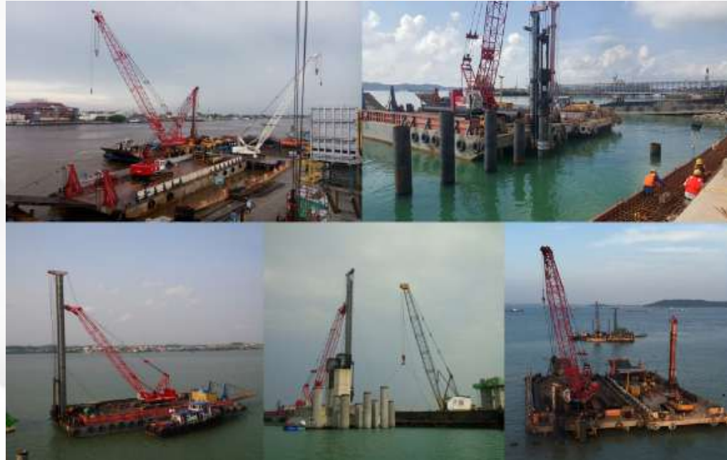
Foundation & Retaining Wall
