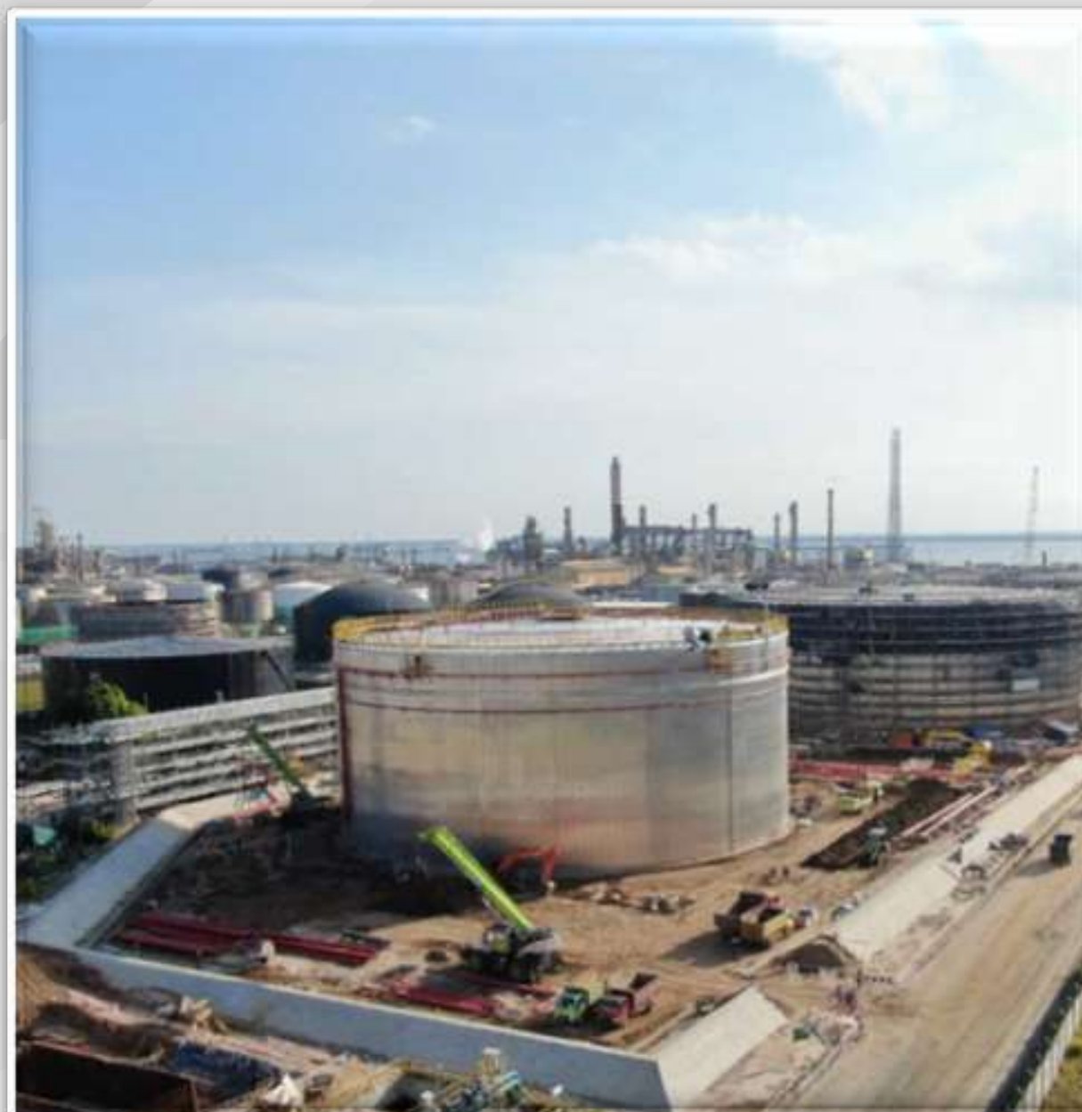
PT RDMP Balikpapan JO Micropile work on the Pertamina Refinery Development Master Plan (RDMP) Project in Balikpapan.
