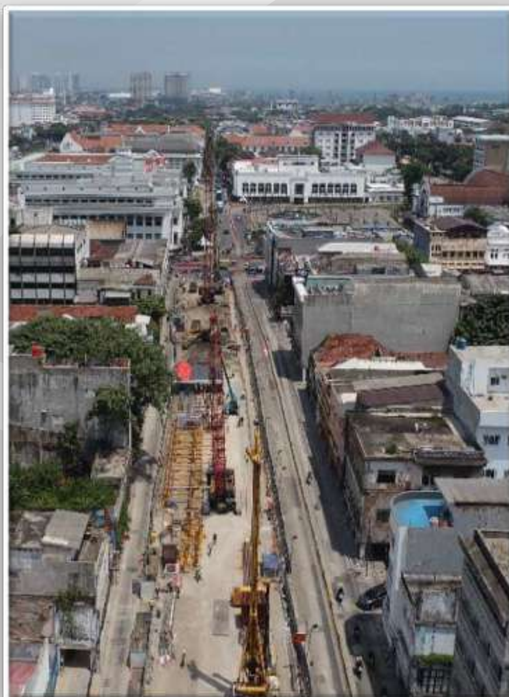
Sumitomo Mitsui Construction Co. PT Hutama Karya Joint Operation Mass Rapid Transit (MRT) Jakarta
