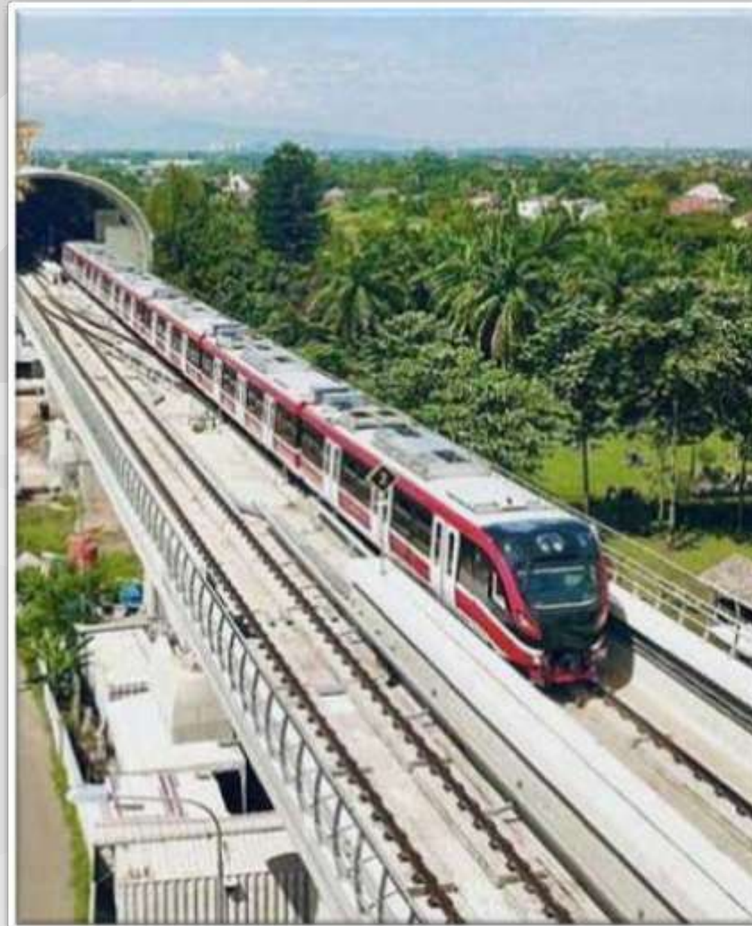
PT Adhi Karya (Persero) Tbk Light Rail Transit (LRT) JABODEBEK
